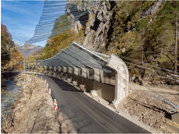
Endzustand Steinschlagschutz Final state of rockfall protection
